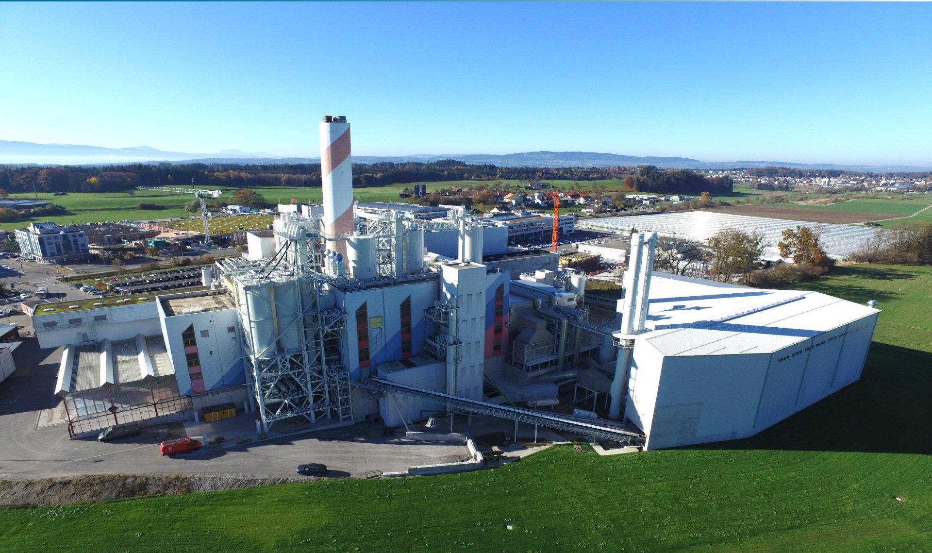
Waste to Energy Plant near the City of Zurich, Switzerland
